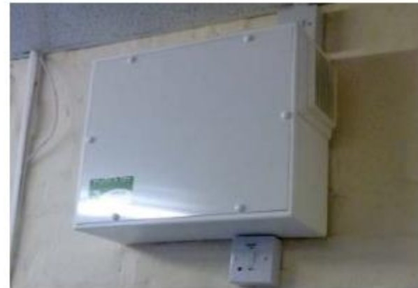
Figure 2: Wall-mounted positive ventilation system
